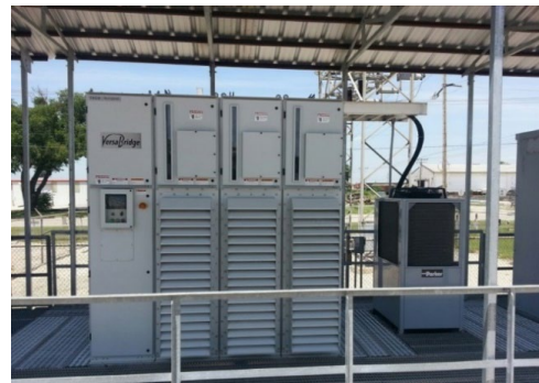
Schematic and actual system installation of a 1 – 2.5 MW SCHB architecture
