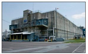
Figure 2-14. SRS's H-Canyon, operational since 1955, contains a processing area 1,028 feet long, 122 feet wide, and 71 feet tall, and is the only hardened nuclear chemical separations plant still in operation in the United States.
