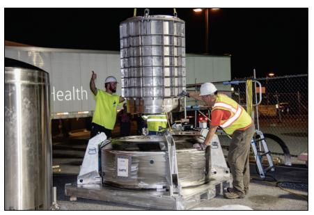
Figure 2-2. ORS and Medstar Georgetown University Hospital worked together to remove a cesium-137 blood irradiator and replace it with an X-ray irradiator at the hospital's Washington, DC, facility.
