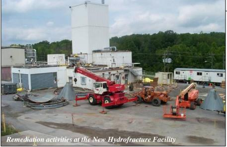
The 107 monitoring wells and four injection wells have been plugged to prevent migration of contaminated fluids to more shallow groundwater zones. The Old Hydrofracture Facility was demolished in 2003. The New Hydrofracture Facility was demolished and waste removed, with the exception of three hot cells. Site restoration was completed in 2006. Groundwater contamination associated with the hydrofracture facilities continues.
