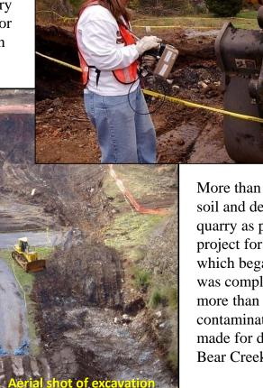
More than 12,000 y<sup>3</sup> of contaminated soil and debris were removed from the quarry as part of the DOE remediation project for ETTP. During the project, which began in November 2004 and was completed in early February 2005, more than 700 truck shipments of contaminated soil and debris were made for disposal at the EMWMF in Bear Creek Valley.
