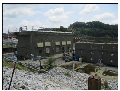
The structure was demolished in early 2010 and the hot cells were encased in a heavy epoxy fixative.
