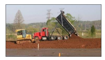
Clean fill being placed over PCB-contaminated sediment
