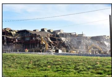
After completing deactivation and demolition activities, building demolition began in February 2016 and was complete in August 2016. The building slab was removed and remedial actions will be completed as necessary to reduce potential hazards associated with contaminated soil.
