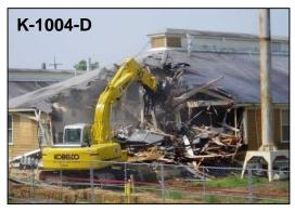
As part of cleanup efforts at ETTP, buildings have been razed at the site at a steady pace and work has been finished on many that were selected for demolition for a variety of reasons: contamination, poor physical condition, proximity to surface water, and surveillance and maintenance costs. These facilities include buildings, tanks, sheds, and other structures. Demolition is accomplished by grouping like facilities into demolition packages to achieve subcontract economies.
