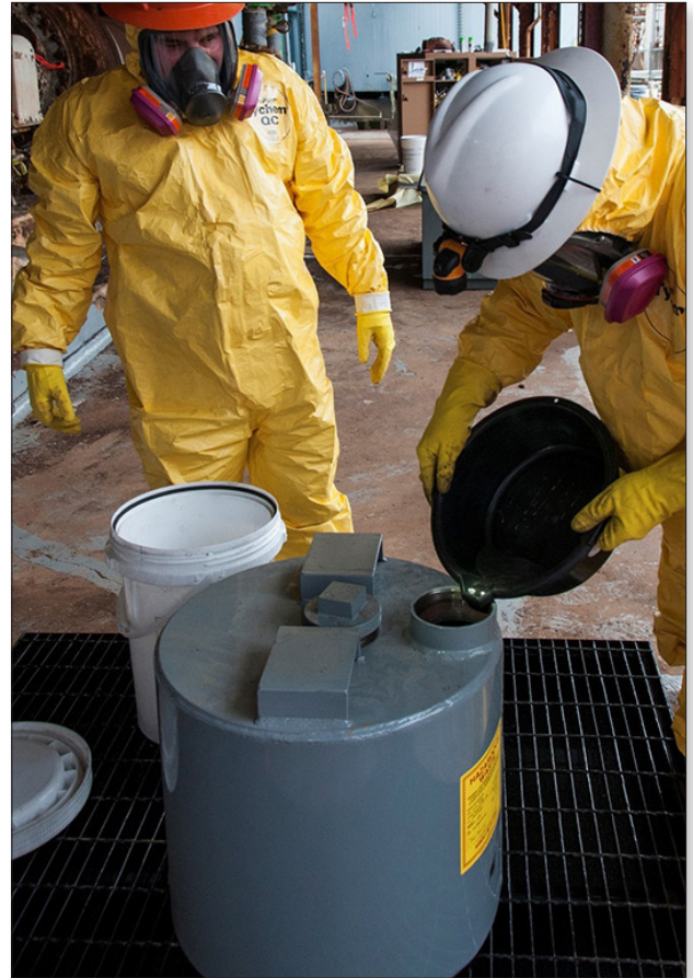
Workers pour mercury from COLEX equipment into a container designed to hold 1,000 pounds of the element.
