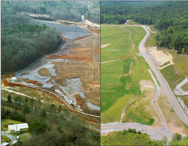
A burial ground area during remediation work, left, and after, right.
