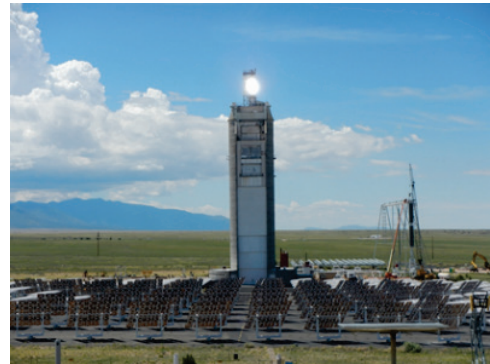
Falling Particle Receiver installed at the National Solar Thermal Test Facility at Sandia National Lab to evaluate proppant (sand-like ceramic particles) as the heat storage medium.
