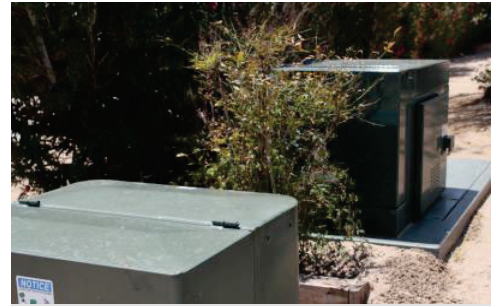
Distributed residential storage for the Borrego Spring MicroGrid—the first of its kind to power an entire community with renewable energy.
