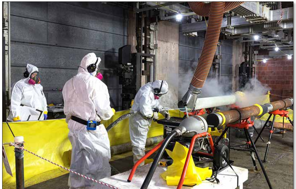
Workers are removing crust and scale from the inside of pipes in the Alpha-4 building.
