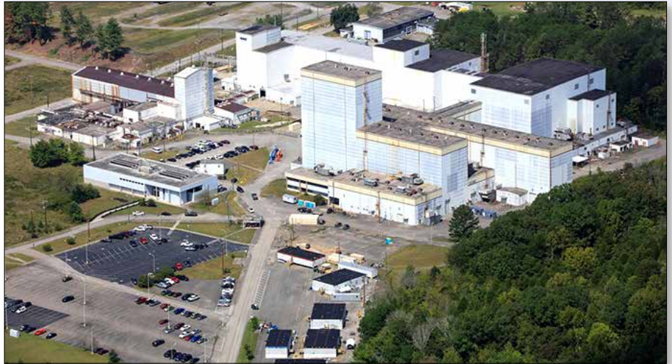
Crews are preparing the Centrifuge Complex for demolition at the East Tennessee Technology Park. EM anticipates beginning the teardown in 2020.
