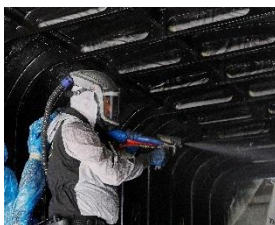
Coating the interior of a 3D-printed house
