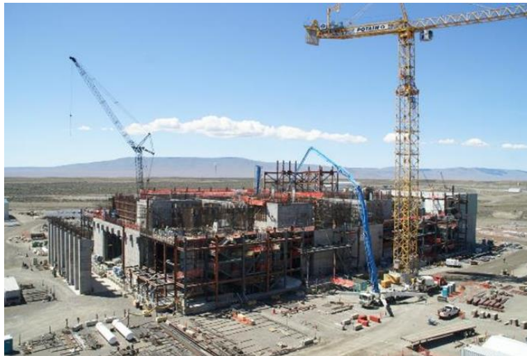
Office of River Protection – Complete construction of the Effluent Management System
