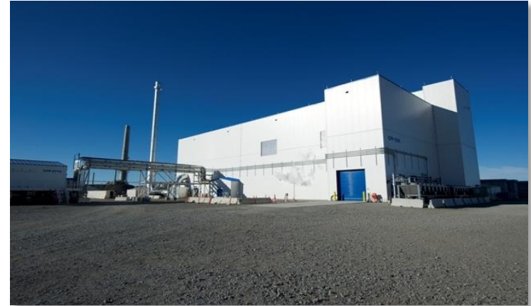
Integrated Waste Treatment Unit
