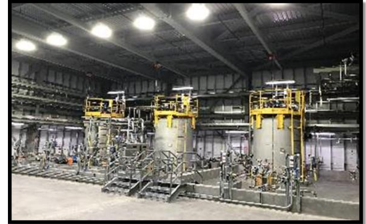
Savannah River Site - Salt Waste Processing Facility Next Generation Solvent Cold Feeds Area
