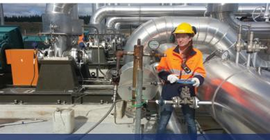
A plant chemist samples silica concentrations from a geothermal injection brine line. Photo credit: Jeff Winick/Allegheny Science and Technology
