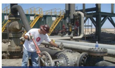
A field engineer setting up well flow test equipment at the Hudson Ranch geothermal power plant in California. Photo credit: Don B. Dale
