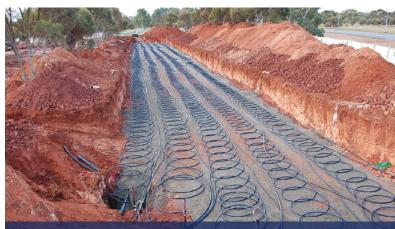
Installation of a horizontal closed-loop ground heat exchanger for a geothermal heat-pump system. Photo credit: Ed Lohrenz/ International Ground Source Heat Pump Association
