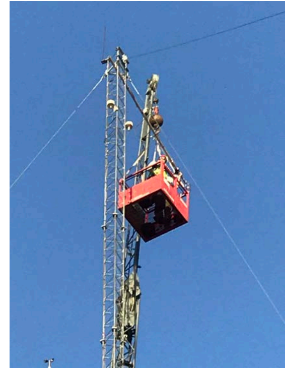
Working with NREL to install Gill Sonic Anemometers on SWiFT met towers - 2018
