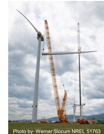
Photo by Werner Slocum NREL 51763
