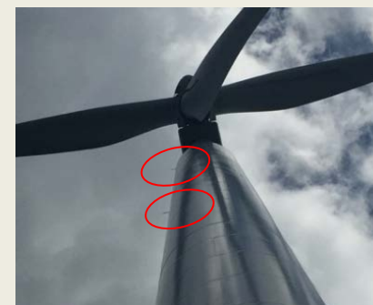
Field Testing of Redesigned Deterrent Installed in Operating Wind Farm
