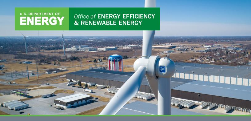
Wind turbines in distributed applications in all 50 states, Puerto Rico, Guam, and the U.S. Virgin Islands provide electricity for on-site consumption or for their local grids. Distributed wind is not defined by turbine or project size, but by a project's location relative to its end use and location on the grid system. This 1.5-megawatt (MW) turbine is one of several that power a Ball Corporation manufacturing facility in Ohio. *Photo Credit: Hank Doster / One Energy Enterprises LLC*
