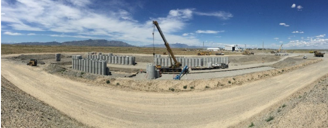
Photo 2: Remote Handled Low Level Waste Project
