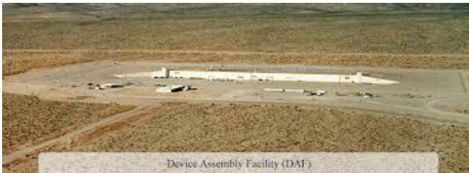
Photo 3: DAF Argus Perimeter Protection Project
