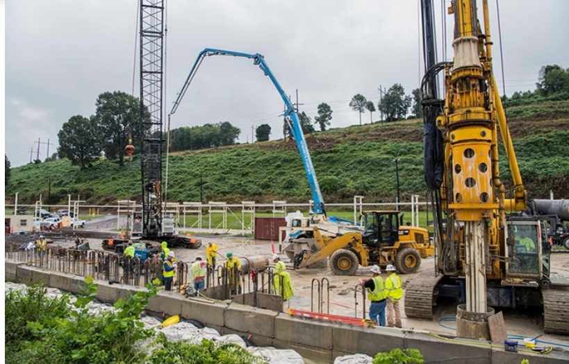
Preparing Site for New Mercury Treatment Facility (OR)
