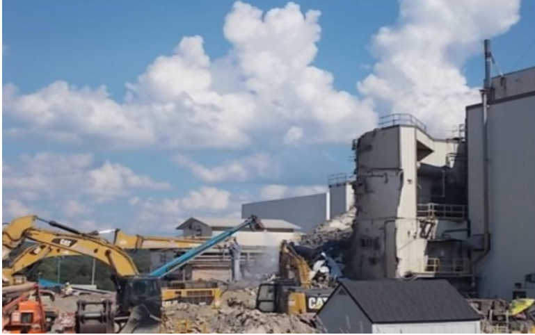
Phase II completion Vit Facility – West Valley
