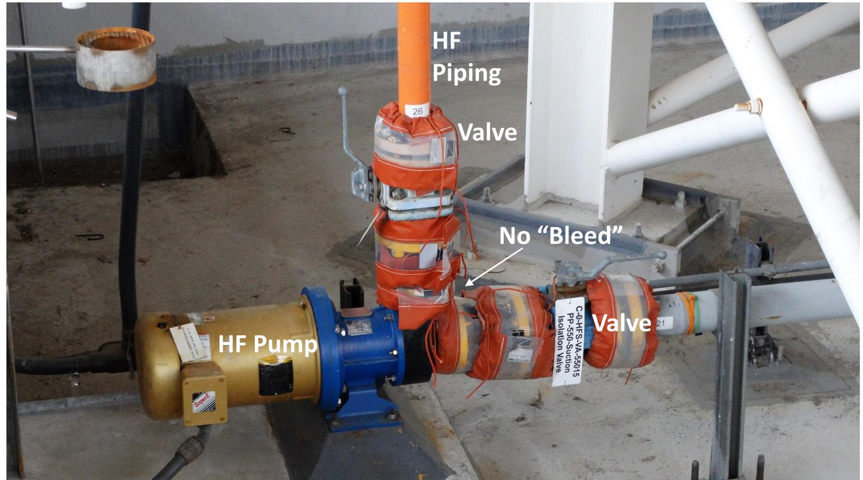
Photo of single block around HF pumps
