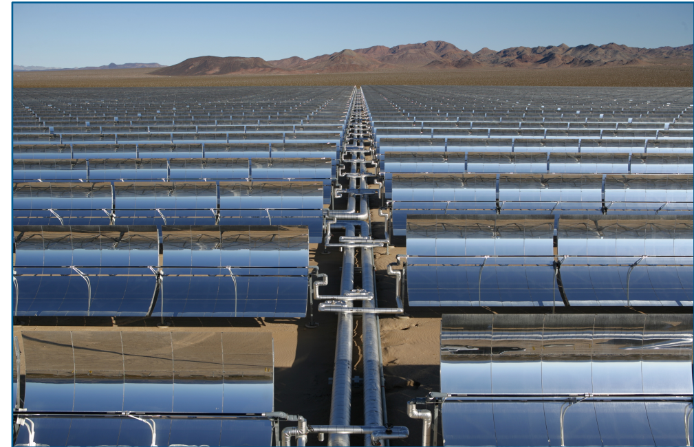
Nevada Solar One Collector Field
