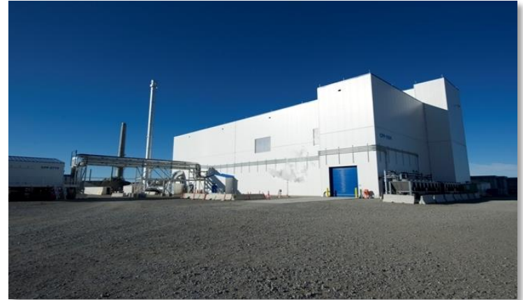
Integrated Waste Treatment Unit
