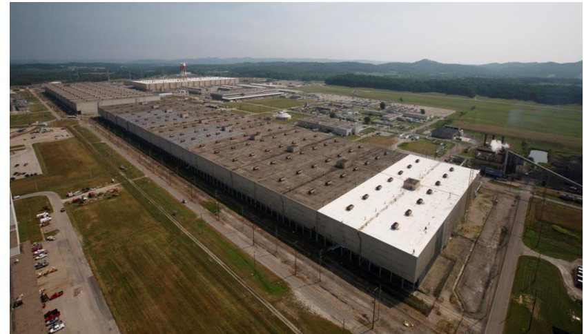
Process Building X-326 at Portsmouth
