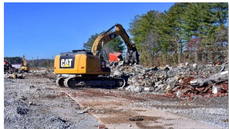
Demolition of East Tennessee Technology Park facilities
