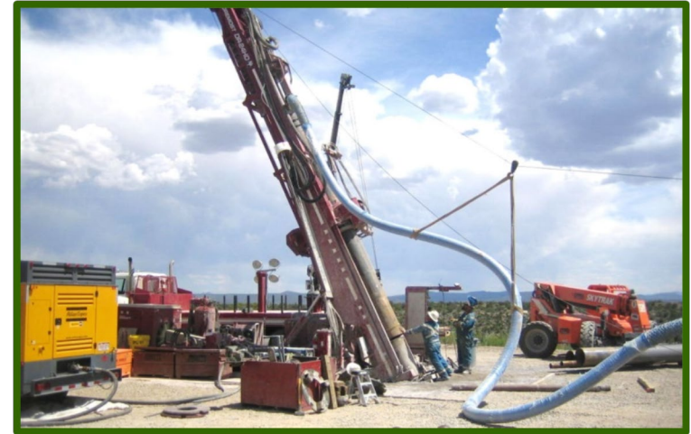
Drilling angled injection well for Interim Measure
