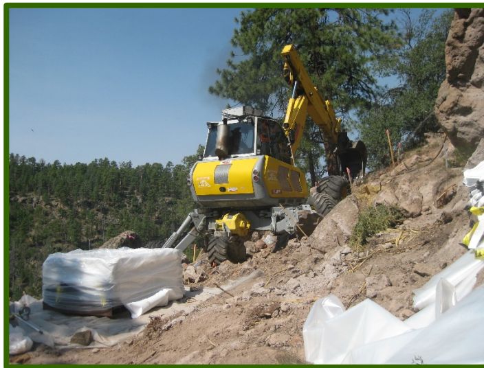
Excavation using a spider excavator at SWMU 01-001(d3)
