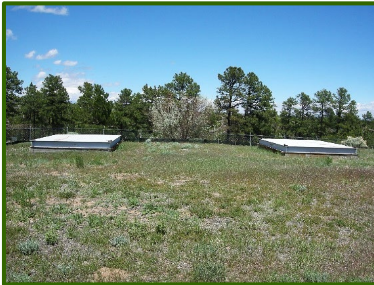
Material Disposal Area A
