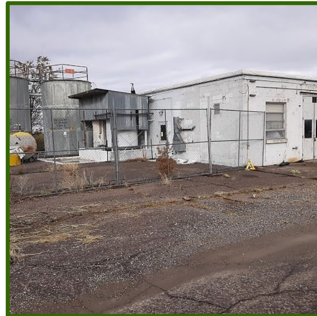
Building 21-257 at Technical Area 21 will be decontaminated and demolished and associated SWMUs/AOCs will be investigated.
