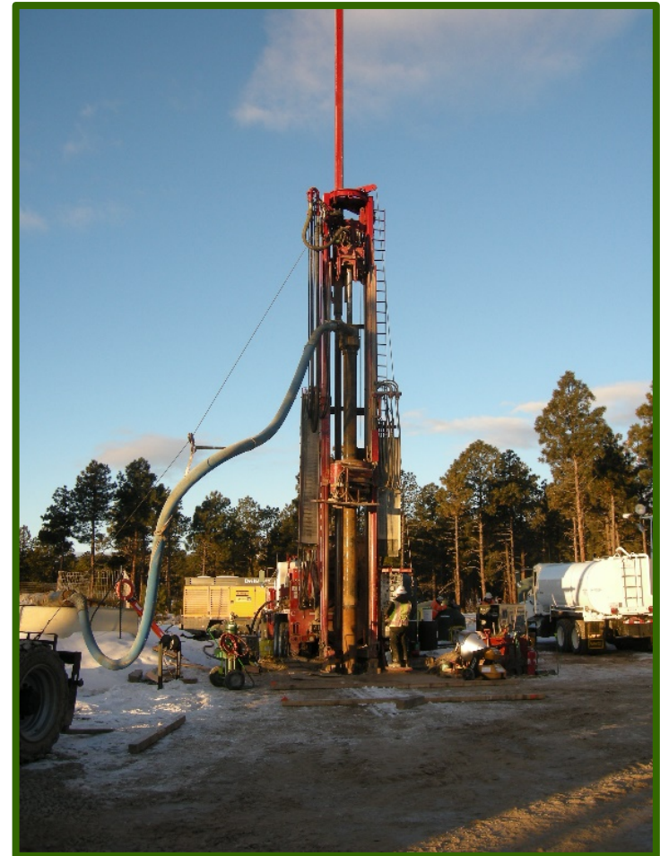
Regional well R-68 under construction
