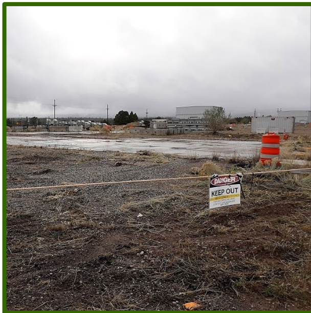
Remaining slabs at DP West at Technical Area 21 will be removed and sumps and waste lines investigated.
