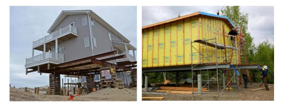
When flood proofing or elevating a building, consider how these changes will increase infiltration or building envelope exposure (e.g., raising a floor will increase the exposed surface area). Energy efficiency measures that can be deployed are weather stripping, air sealing, and increasing the R-value of insulation.
