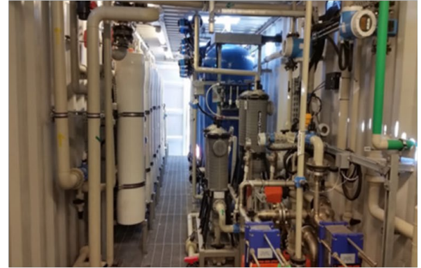
PC Membranes, Pre-treatment and Heat Recovery HX
