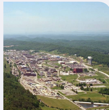
Y-12 National Security Complex
