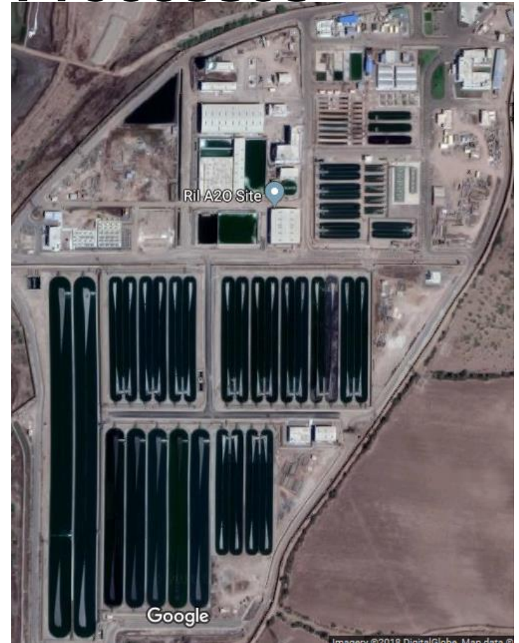
Image of RIL Gagwa facility. Longer ponds on left are over 1 km long. Includes harvesting, HTL, media mixing, central control room. Refinery nearby.
