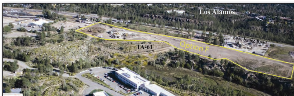
Figure 5.1-4. Brownfield site at the capped County landfill (TA-61)
