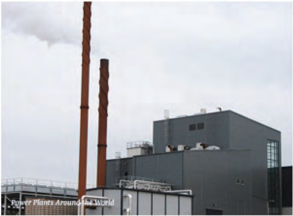
Picture 3: 5.3 Megawatt wood fired Combined Heat and Power plant
