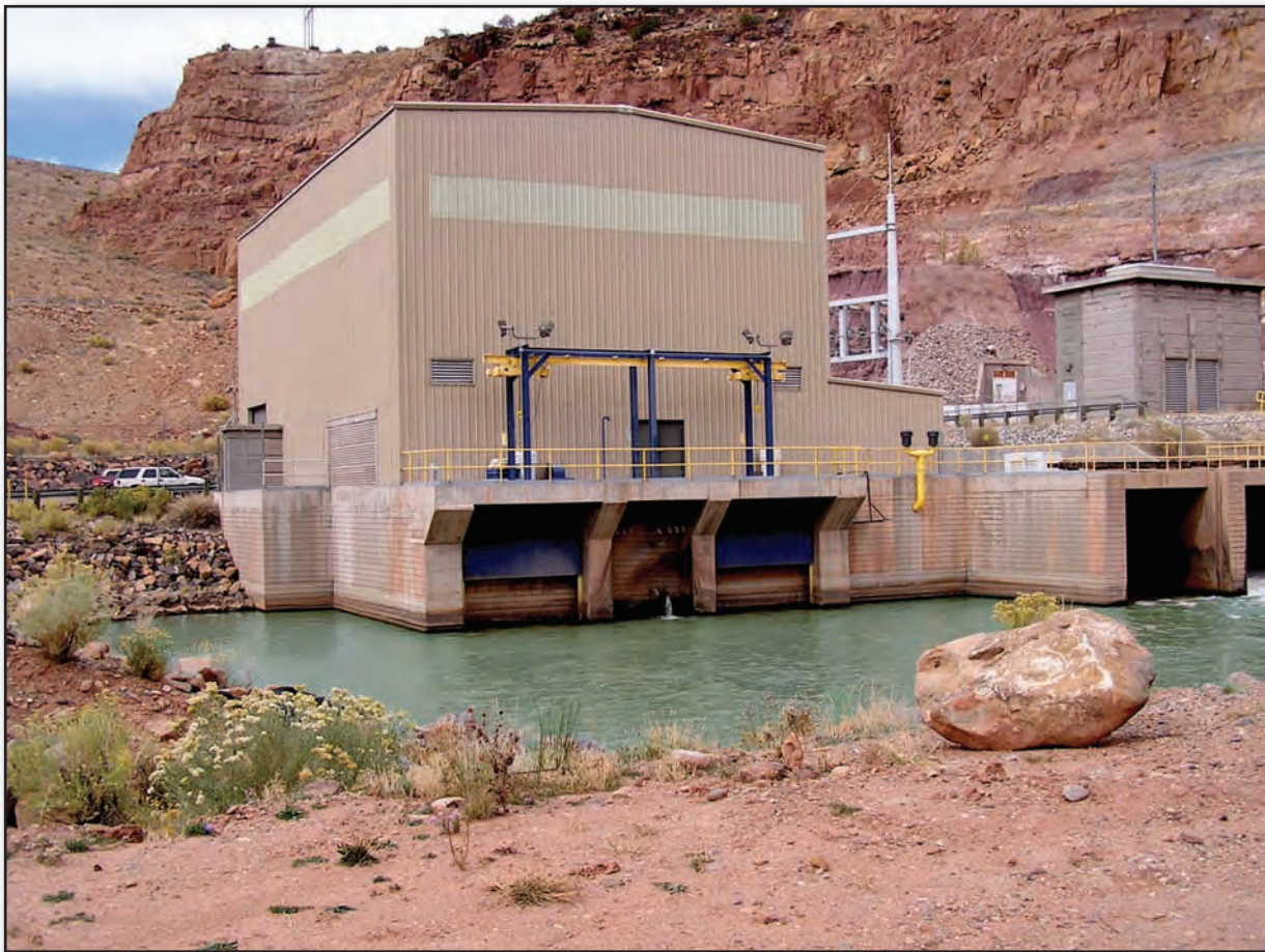
Figure 5.7-1. Abiquiu Dam hydroelectric plant (Los Alamos County Department of Public Utilities).
