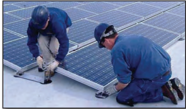
Figure B-7. Roof mounted 700 kW PV system, Shisheido America HQ (Sunpower Corporation).
