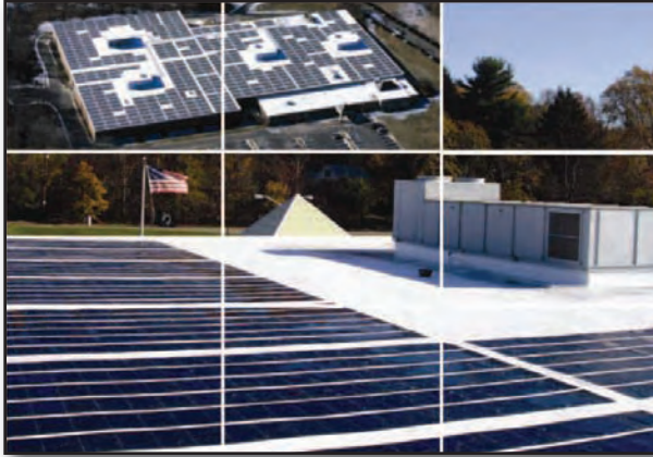
Figure B-5. PV integrated roof installation (Silka Sarnafil, Inc. and Solar Integrated Technologies).
