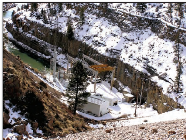
Figure A-1. El Vado Hydroelectric (Los Alamos Department of Public Utilities).
