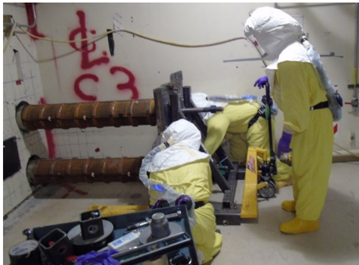
Workers training in a mock-up facility prepare to dig highly contaminated soil out from under the 324 Building.
