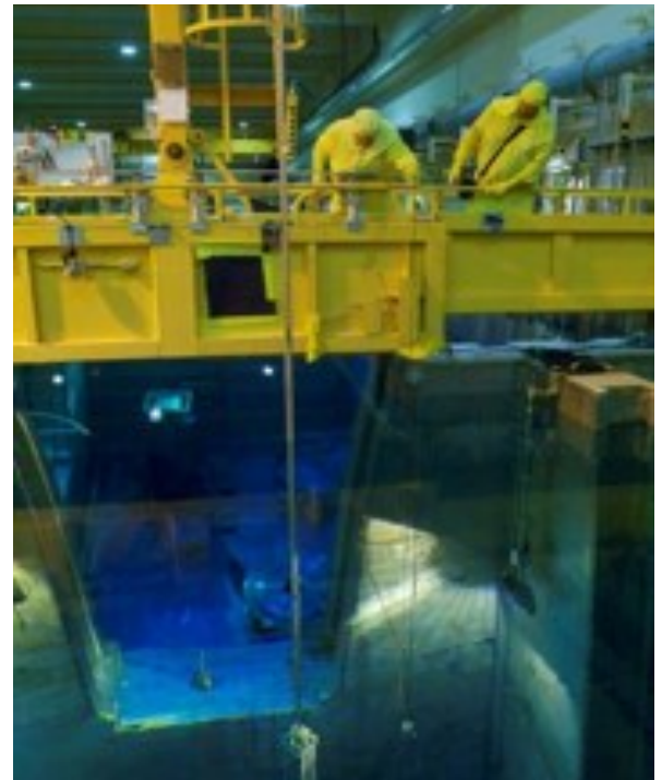
Workers extract spent nuclear fuel from the CPP-666 spent fuel basin as part of a project to move all spent fuel from wet to dry storage.
