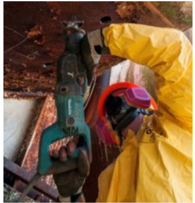
Workers retrieved more than 6,000 pounds of mercury from the COLEX equipment's tanks and pipes.
