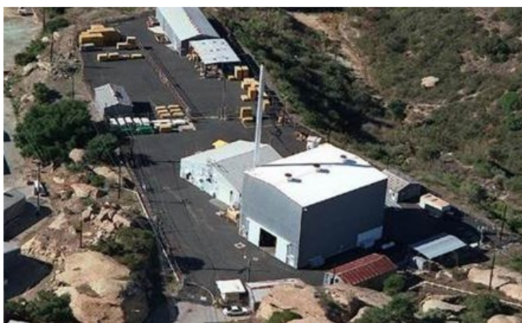
Radioactive Materials Handling Facility.
