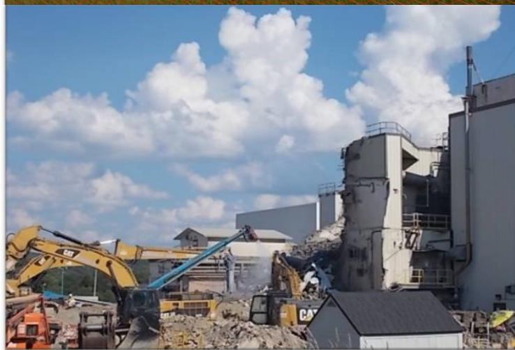
WVDP Vitrification Facility—Before and After.
