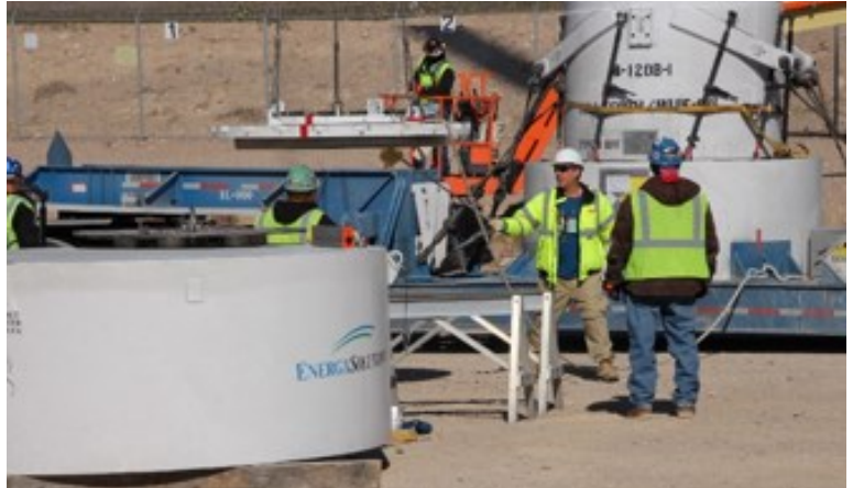
A radiological control technician surveys a cask lid before workers proceed with removing waste packages for disposal.
