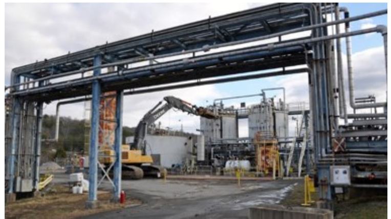
Teams took down the Central Neutralization Facility.
