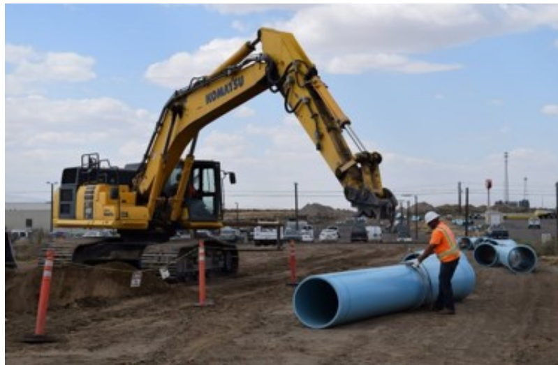
Workers maintain and upgrade infrastructure systems across the site.
