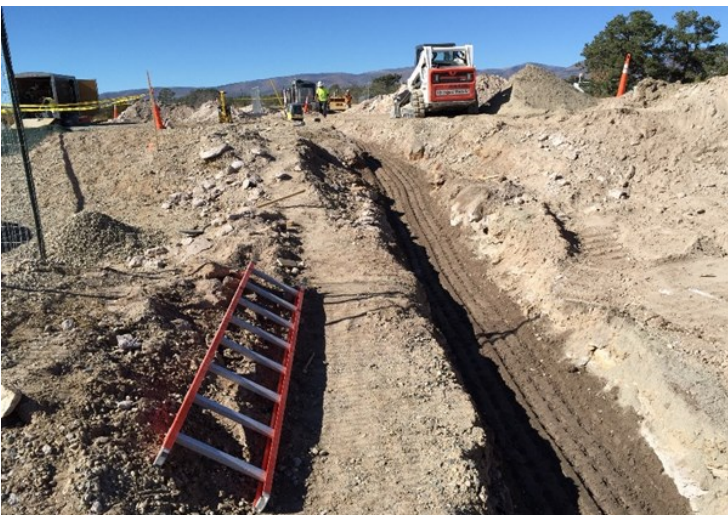
Over three miles of pipeline were installed in 2018 for Chromium Interim Measure and Characterization Campaign.
