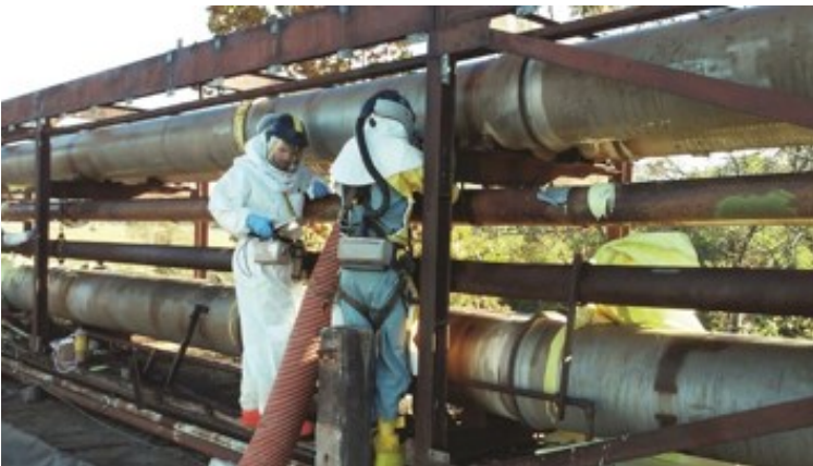
Workers finished removing all four miles of tie lines at ETPP.
