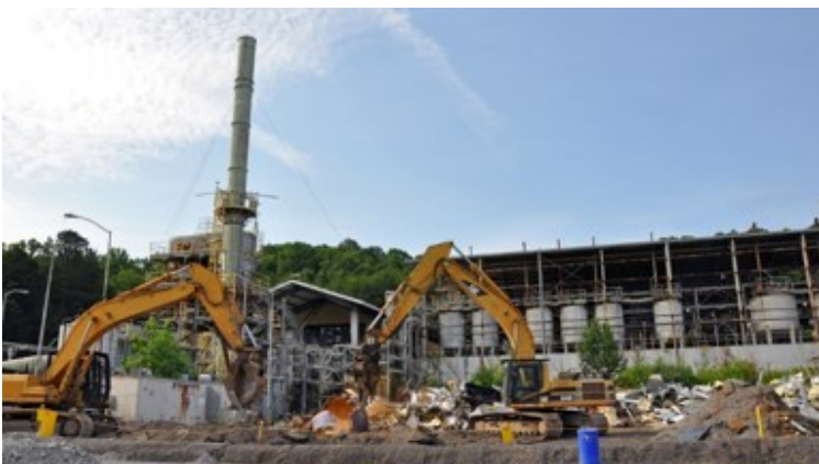
Workers demolished the TSCA Incinerator.
