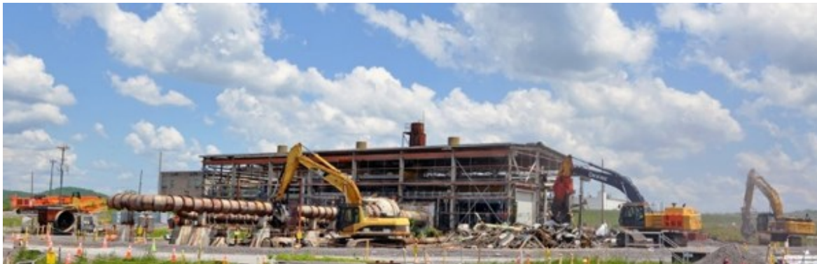
Crews demolish Building K-633 in the Poplar Creek area.
