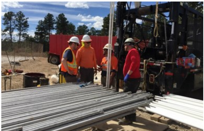
Workers review safety procedures prior to groundwater sampling system installation.
