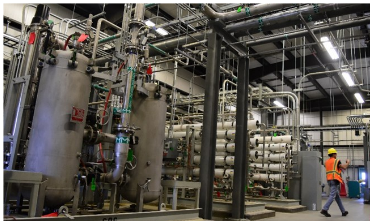
The Water Treatment Building is one of five WTP support facilities that have been handed over for commissioning.
