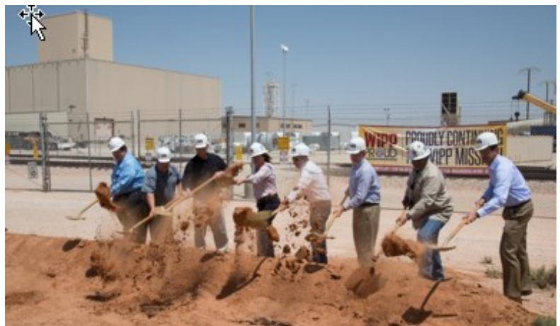
EM Assistant Secretary Anne White, fourth from left, participates in the June 14 groundbreaking for the Safety Significant Confinement Ventilation System.
