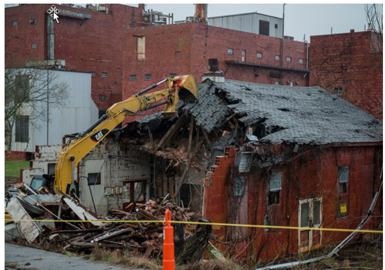
Removal of two high-risk excess contaminated facilities in Y-12’s Biology Complex.
