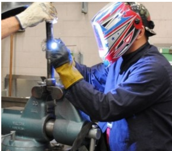
Savannah River Remediation employee safely completes welding work at the Defense Waste Processing Facility.
