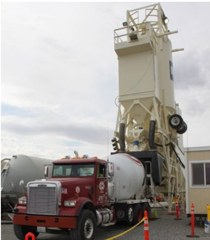
Workers began filling PUREX No.2 waste storage tunnel with engineered grout.
