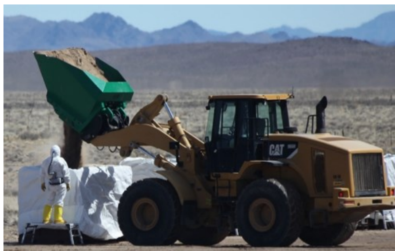
Contaminated soil is packaged at the Clean Slate II site.
