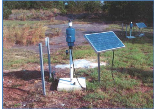
Solar energy provides power to microblower that removes volatile contaminants from beneath the ground surface
