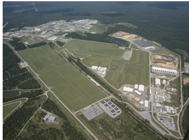
E-Area Waste Storage and Disposal Facilities
