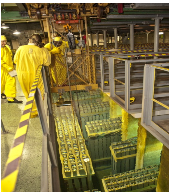
Spent Fuel Storage in the L-Area Complex
