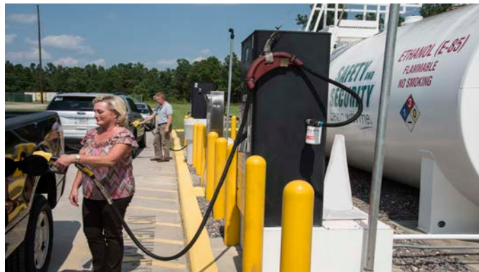
E85 fueling station provides fuel for Site vehicles
