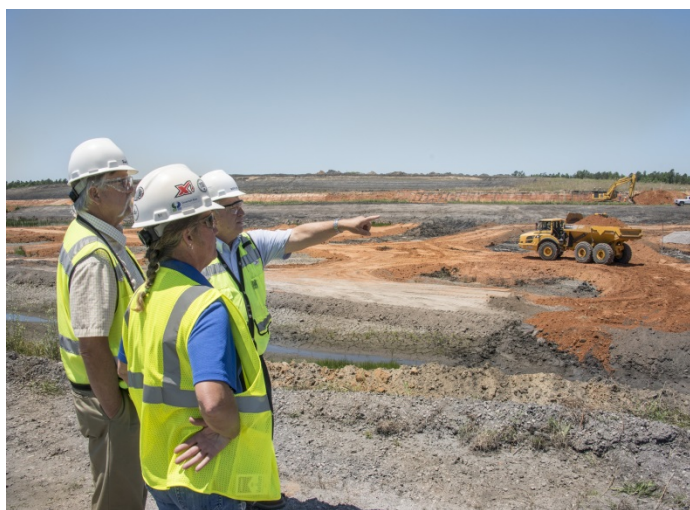
SRS Employees Observe D-Area Coal Ash Basin Closure Activities
