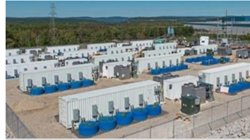
20-MW flywheel facility in Hazle, Pennsylvania
