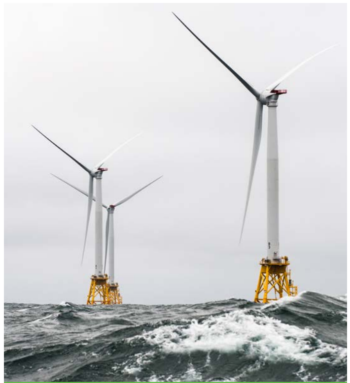
The Block Island Wind Farm, the first U.S. offshore wind farm, represents the launch of an industry that has the potential to contribute significantly to a clean, affordable, and secure energy mix. Photo by Dennis Schroeder, NREL 40389
