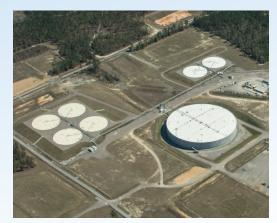
SDUs 2,3, and 5 (3 and 5 pictured left) are cylindrical tanks that are 150 feet in diameter, 22 feet tall, and hold approximately three million gallons of grout each. SDU 6 (pictured below), SRS's first mega-volume SDU is a cylindrical tank ten times larger than previous SDUs. SDU 6 construction was completed in July 2017. SDU 6 is 375 feet in diameter, 42 feet high, and will hold approximately 32.8 million gallons of grouted decontaminated low-level salt waste.
