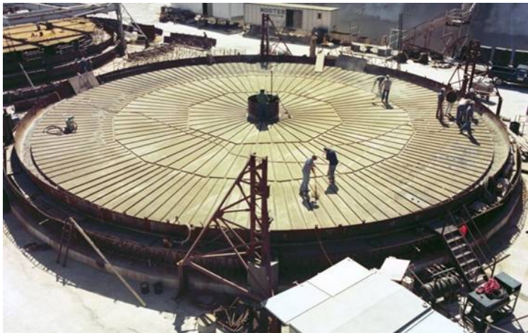
Figure 2.1-46: Typical Type III/IIIA Tank Radial Air Grooves
