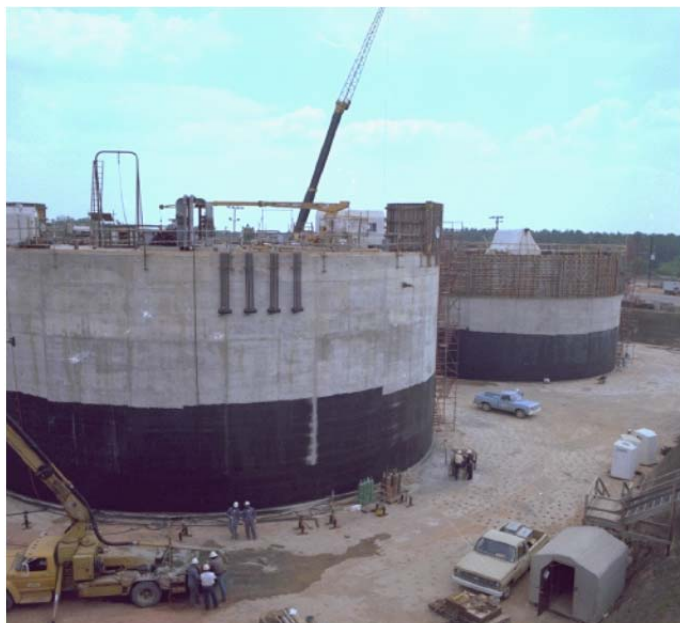
Figure A.2-1: Waste Tanks Under Construction
