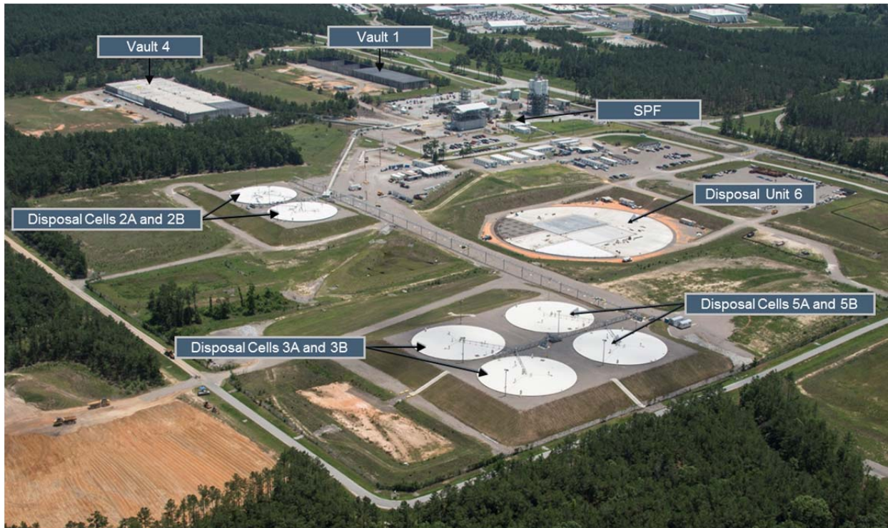
Figure A.3-3: Saltstone Facility (June, 2014)
