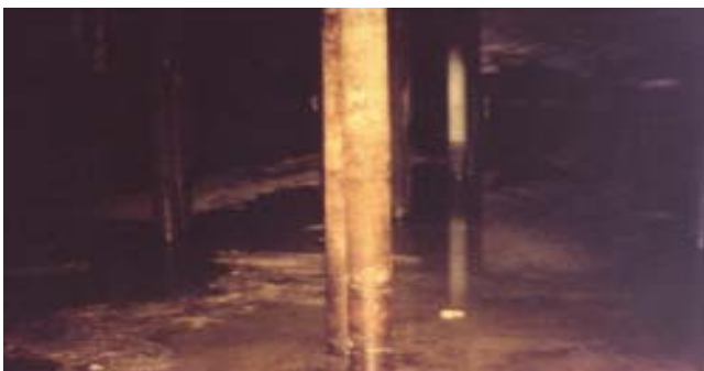
Figure A.2-2: Supernate (Top) and Saltcake (Bottom)
