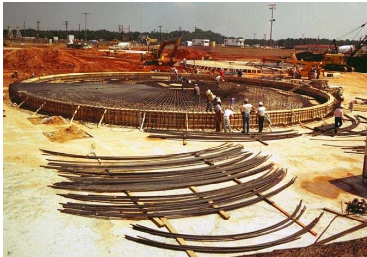
Figure 2.1-44: Typical Type III/IIIA Tank Basemat Construction
