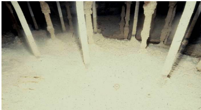
Figure 2.2-1: Saltcake at Bottom of Waste Tank
