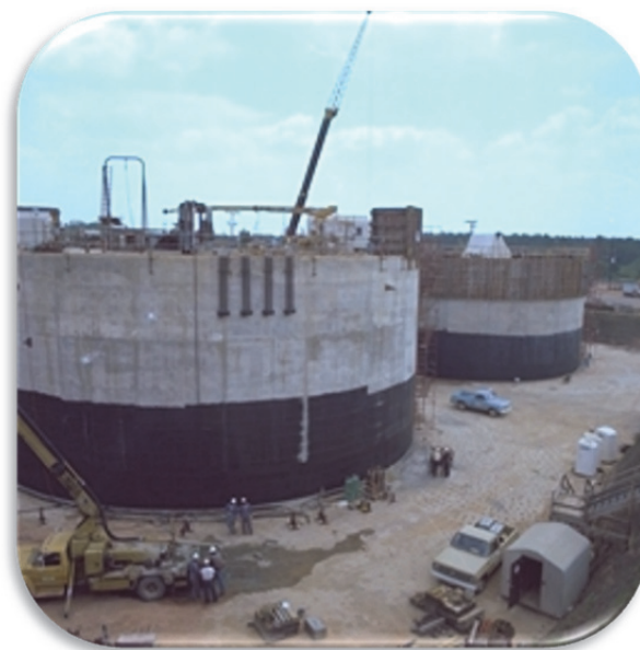
Tanks under construction. Note tank size relative to construction workers. Later, dirt is backfilled around the tanks to provide shielding
