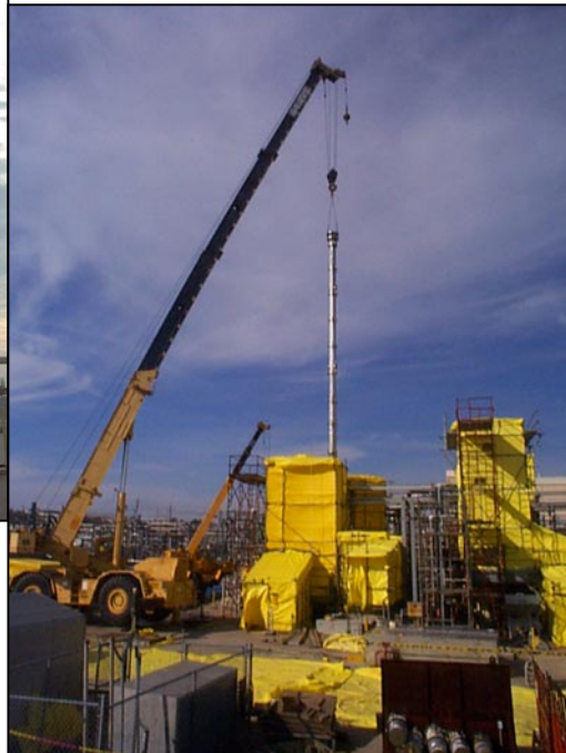
Typical Waste Removal equipment includes three to four 45-foot long slurry pumps and one transfer pump or jet. Note the substantial structural steel required to support the loads in the picture above. At right is the typical installation of a transfer pump (Tank 8) requiring difficult, high-risk entries into High Level Waste Tanks.
