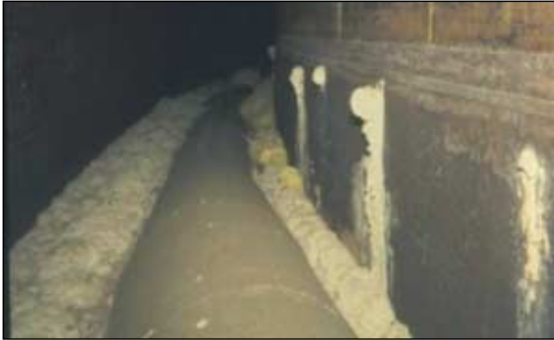
Tank Annulus showing High Level Waste that has leaked from the Primary Tank in the past and has solidified
