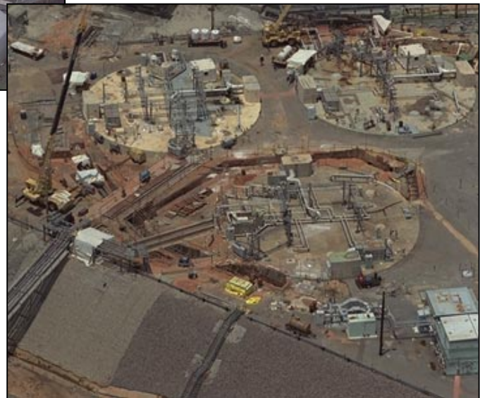
Overhead View of H Tank Farm showing the tops of three tanks. Each tank is approximately 90 feet across and can contain over one million gallons of waste.
