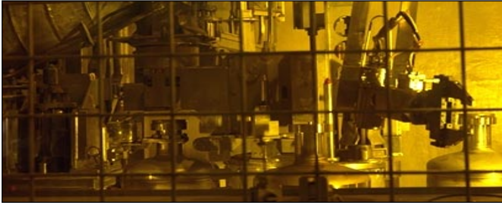
View through protective shielding of DWPF Melter Cell showing a canister being filled.
