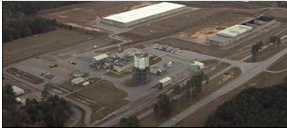
View of Saltstone Facility: Processing Facility in foreground, two vaults in rear.
