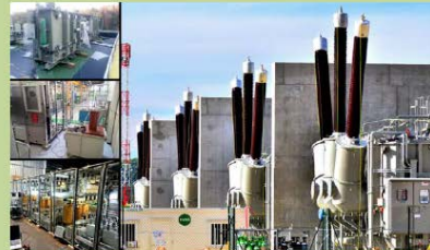
US completed delivery of Steady State Electrical Network components to the ITER site in 2017.
