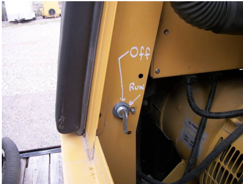
Figure 2. Battery Isolation Switch
