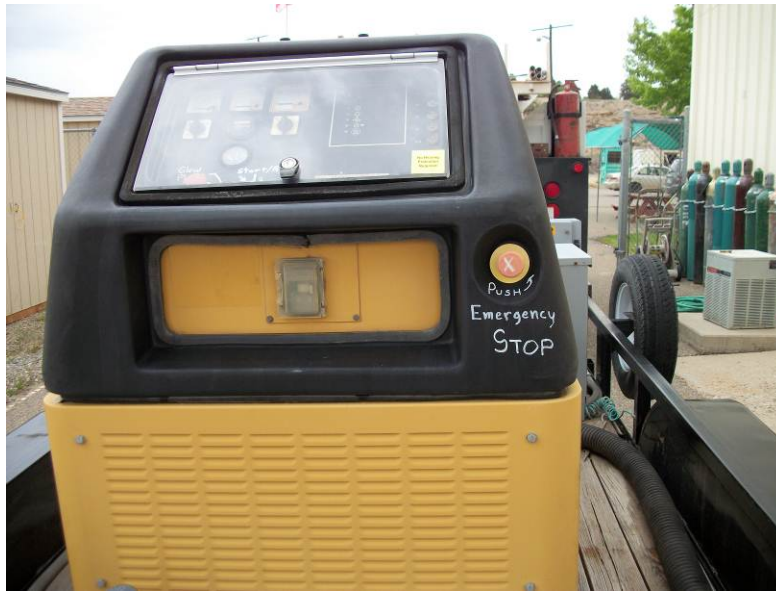
Figure 5. Emergency Stop Button
