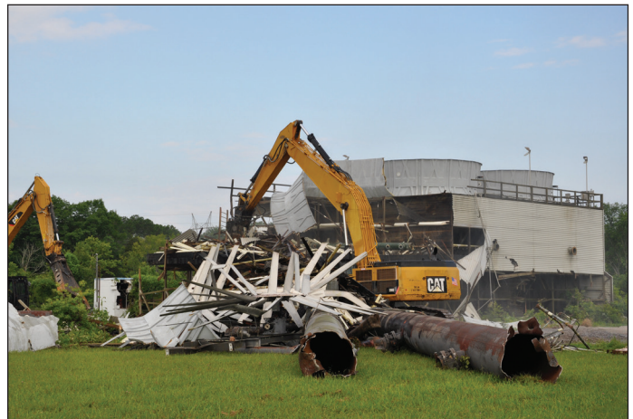
K-832-H Cooling Tower demolition
