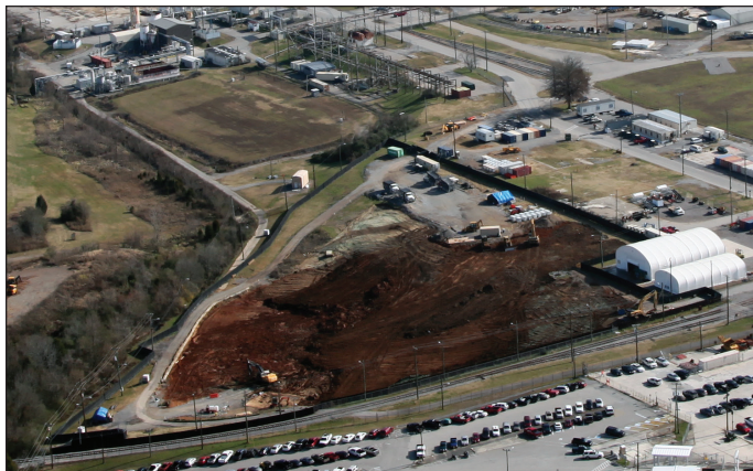
K-1070-B during remediation
