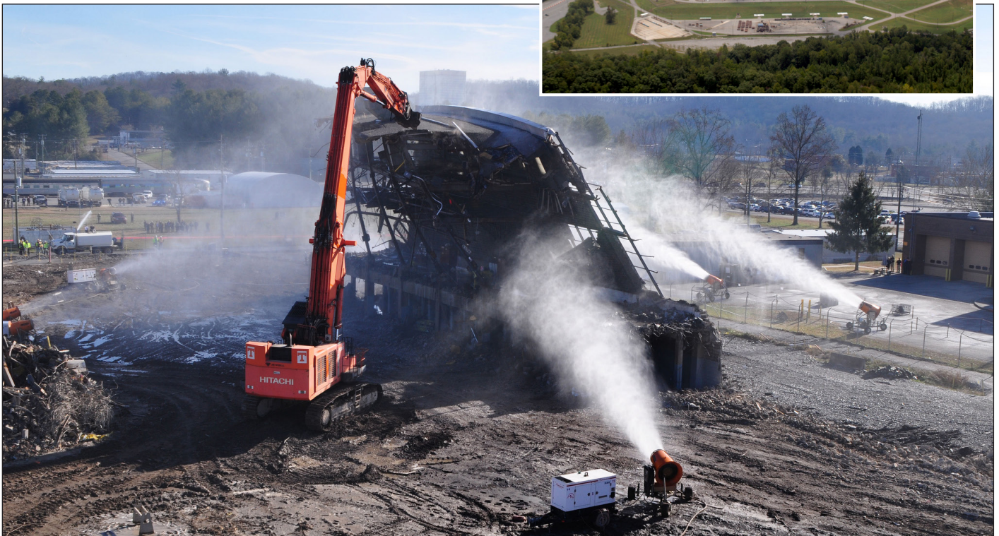
The final section of the K-25 Building was demolished in December 2013.
