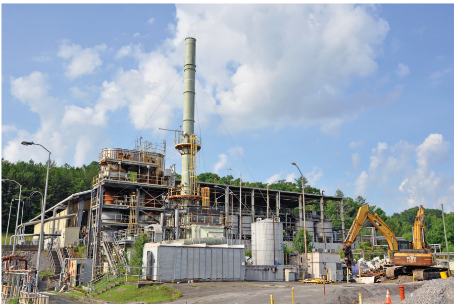
Demolition of the TSCA Incinerator
