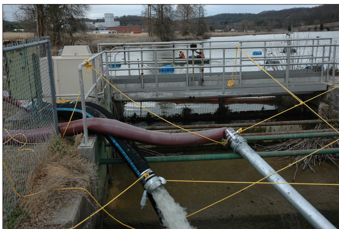
One of the contaminated ponds at ETPP being drained
