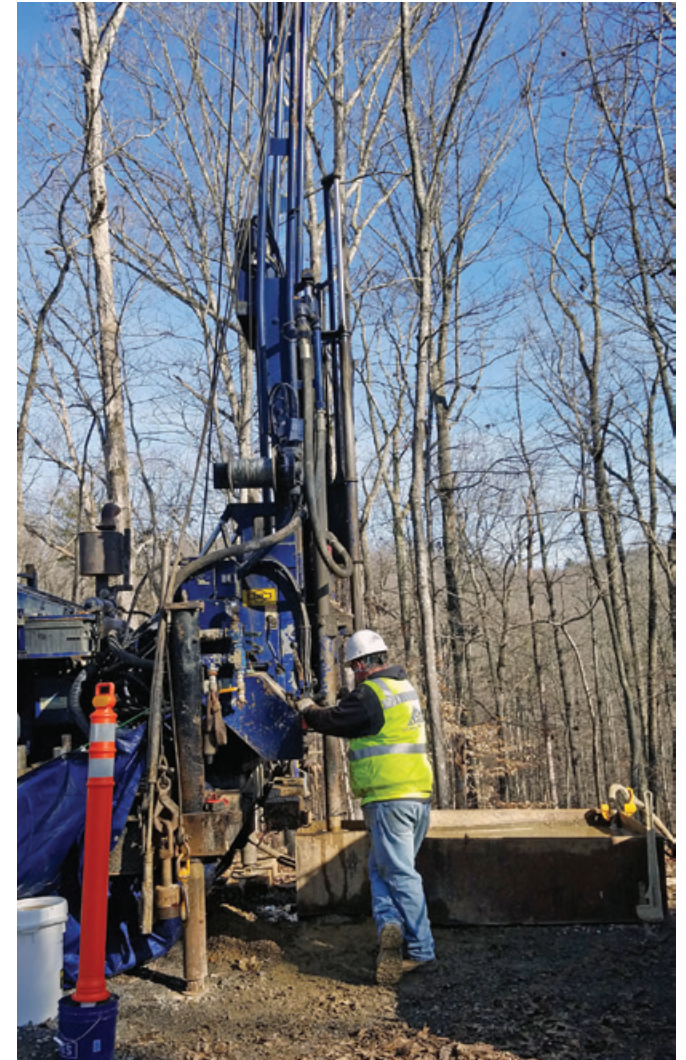
Well installation at the proposed EMDF site
