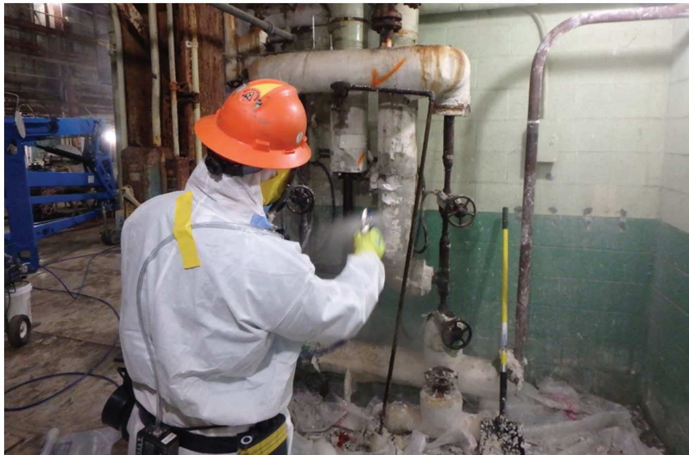
Pipe insulation removal in Building 7500
