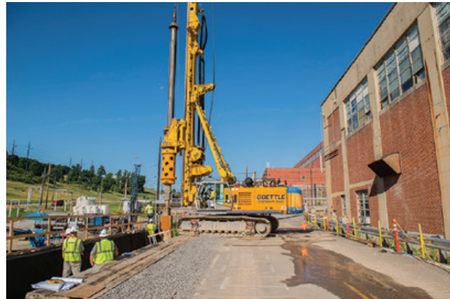
Workers install the north secant pile wall, which serves as a retaining structure.
