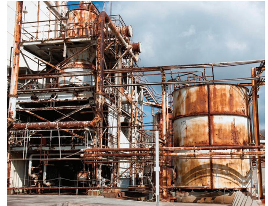
COLEX facility before demolition activities
