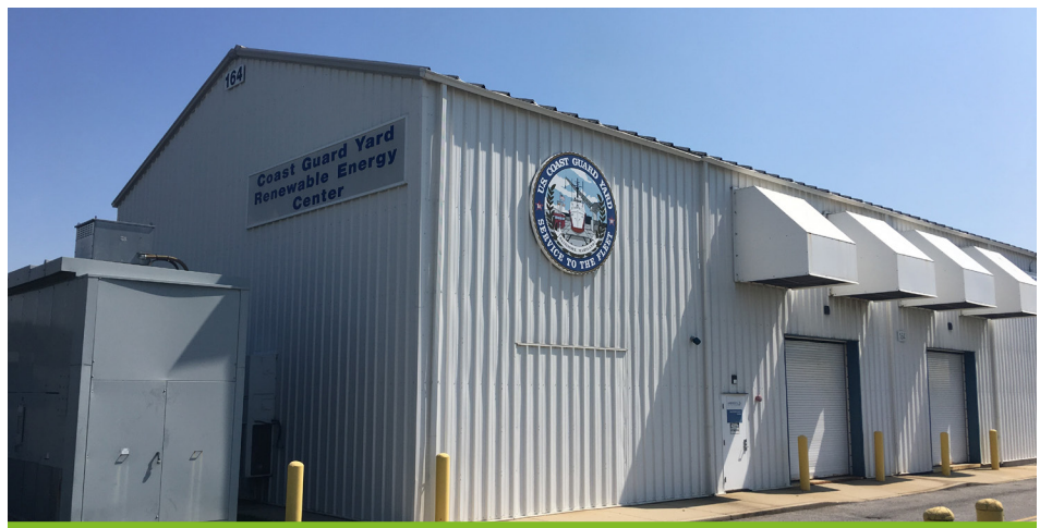
Coast Guard Yard Renewable Energy Center Photo courtesy of U.S. Coast Guard.
