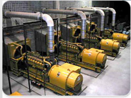
Existing Diesel Generators (6 MW)
