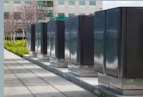
Fuel Cells (1 MW scalable)
