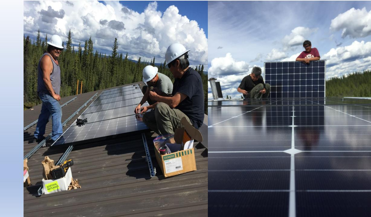
After Final Install of all solar arrays A contract electrician and TCC energy completed final hook up and activated two of the three systems the 3<sup>rd</sup> system had a bad rapid shut down and required replacing. Alaska Power and Telephone came and installed new meters
