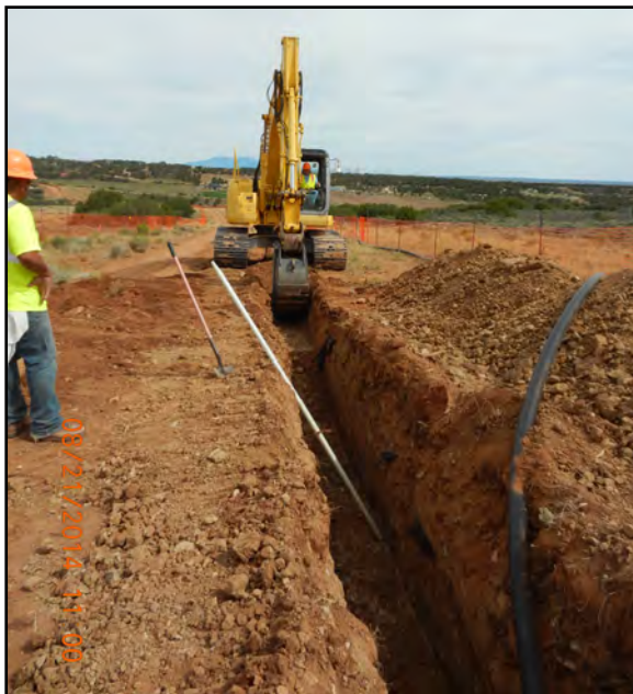
Workers excavate a trench to bury a sub-grade pipeline that allows the groundwater treatment system to operate year round.
