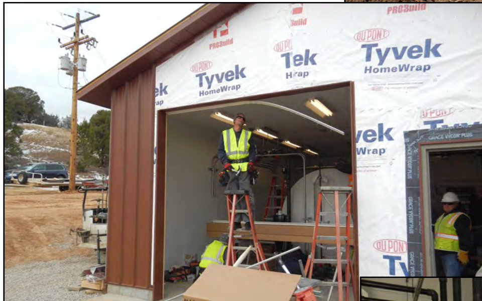
A groundwater transfer building holds an aboveground batch tank that collects extracted groundwater. A strong pump on the tank sends the water to the evaporation pond on LM property.
