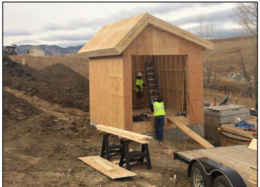
Figure 3. The new, commercial air stripper is shown in the left photo above, and will be housed in the shed shown in the photo on the right. The roof of the shed is angled to provide better solar-thermal exposure. The solar/battery conex from Figure 2 (see page 14) is visible in the background to the left of the shed.
