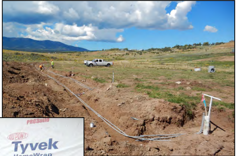
Conduit was installed to house electrical control and well field components.
