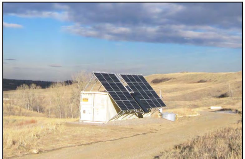
Figure 2. Air stripping at the East Trenches Plume Treatment System focused on water that was not yet treated using iron filings. The spray nozzles (above left) are located in the gray manhole next to the solar array shown in the photo on the right. The solar panels charge batteries located inside the conex, which power the pump.
