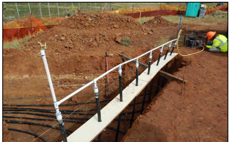
Piping from eight extraction wells is pressure tested to ensure it meets specifications.
