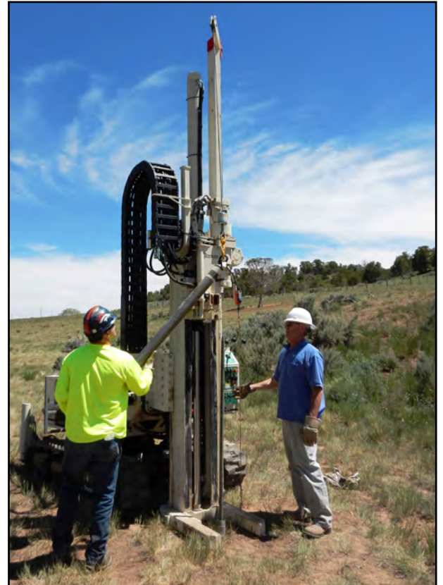
Workers install new monitoring wells to track progress of the remedy optimization.
