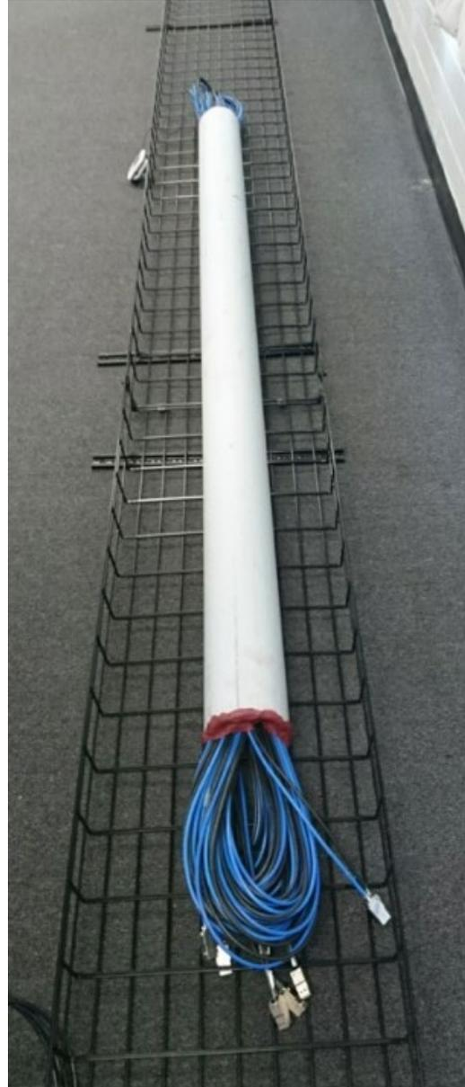
**Figure 8. Cable bundled in Schedule 40 PVC conduit, prior to connecting the field-terminated jacks to the patch cords with factory-terminated plugs.**
