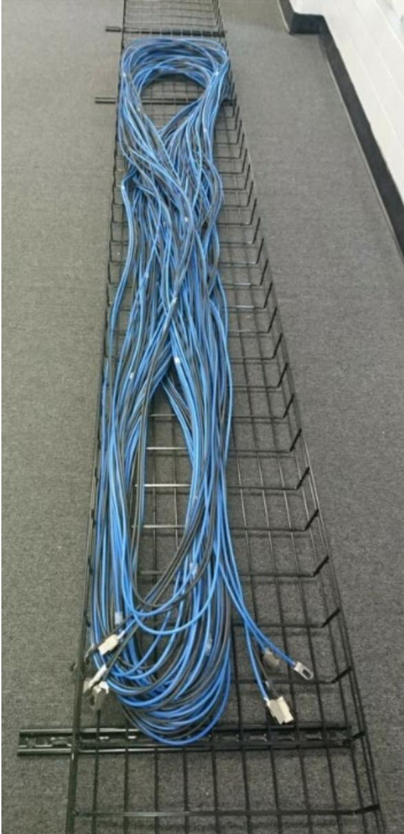
**Figure 7. Cable loose in cable tray (not bundled), prior to connecting the field-terminated jacks to the patch cords with factory-terminated plugs.**
