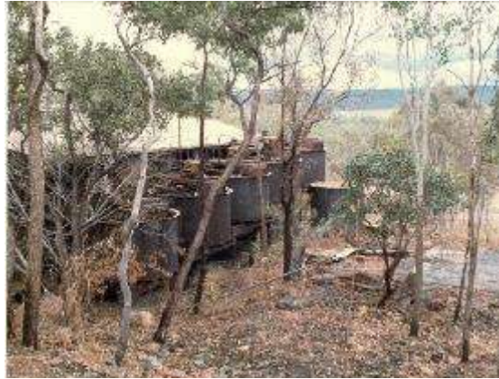
SAV Mill, near Rockhole mine
