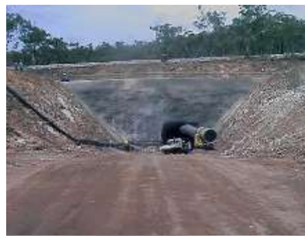
1998 – Portal & decline construction
