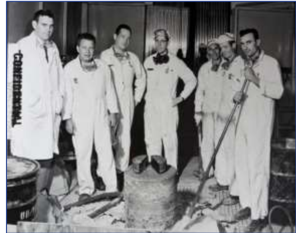
Weldon Spring Uranium Feed Materials Plant AEC, 1957-1966
