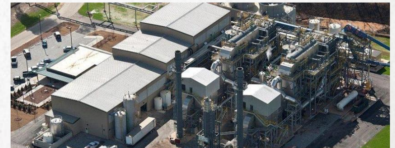
SRS Biomass Facility
