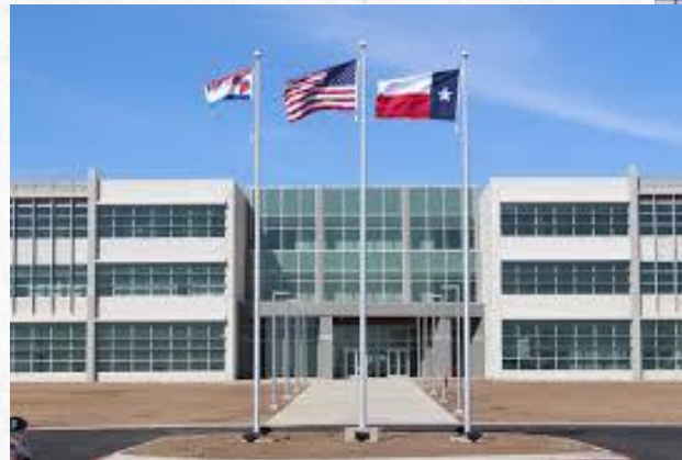
Pantex New Administrative Building
