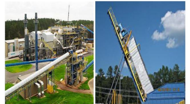
SRS Biomass Cogen Plant
