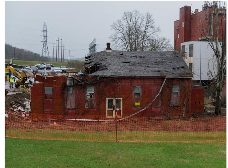
Y-12 Biological Facility Progress
