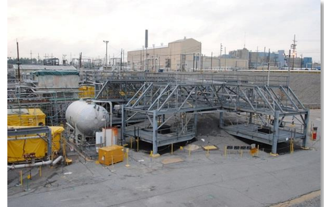
Tank 20 at the Savannah River Site
