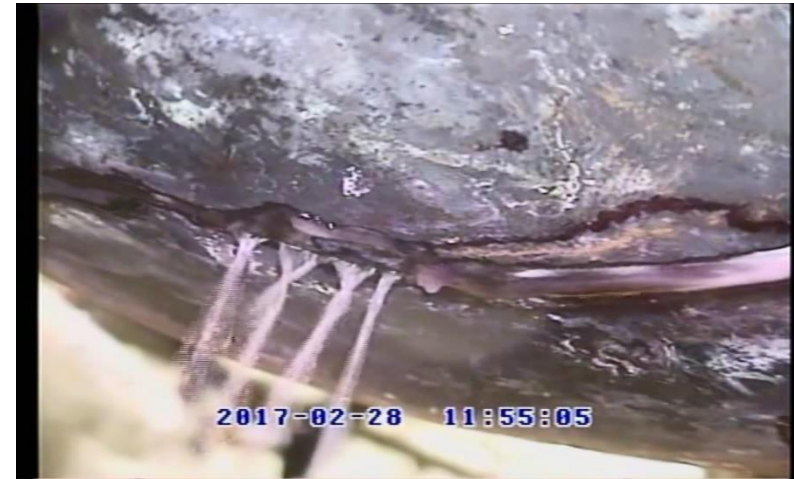
SRS 3H evaporator leak
