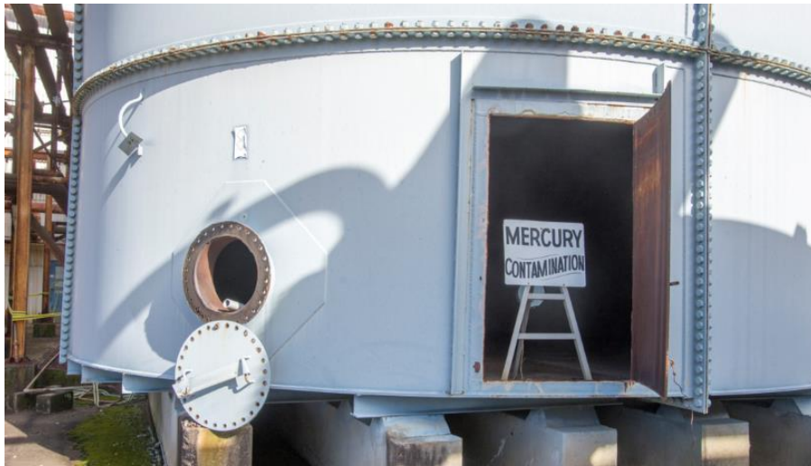
COLEX Equipment at Y-12
