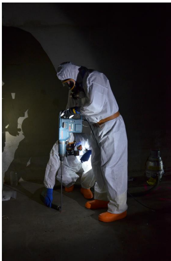
Figure 3.2. Installation of Vapor Intrusion Sampling Port
