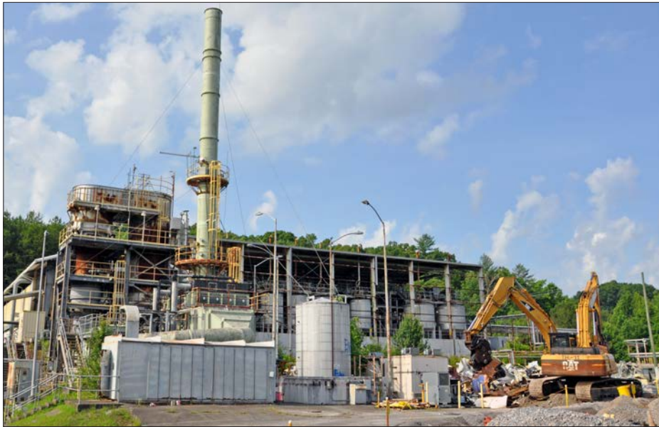
Initial demolition activities at Oak Ridge's TSCA Incinerator began this summer.
