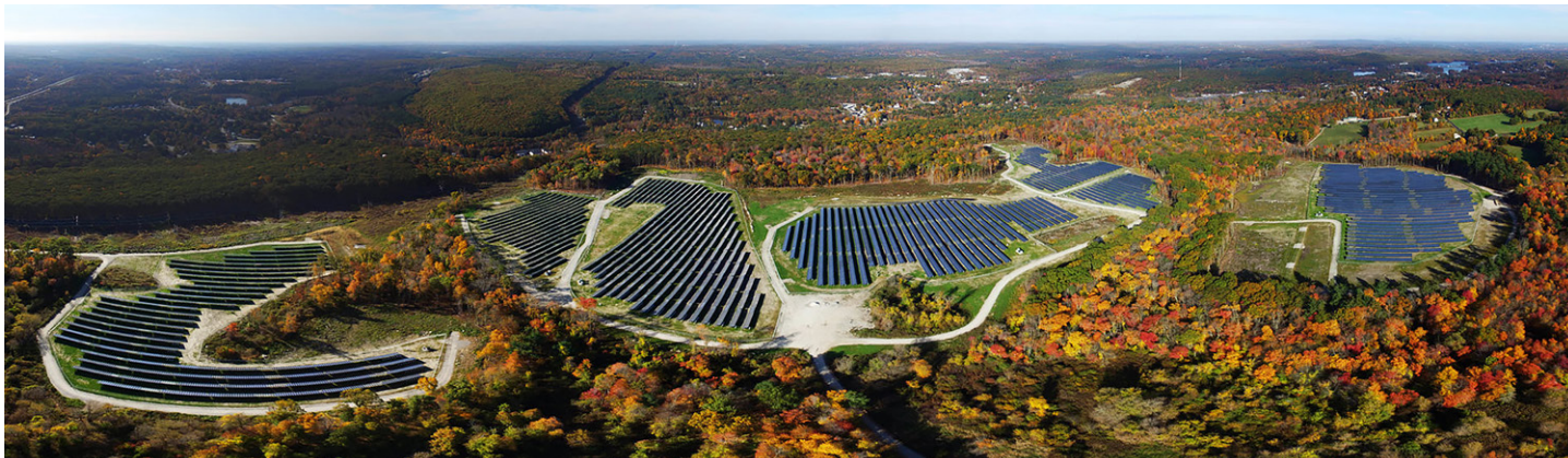
This 16.5 megawatt solar farm was built on a 130-acre property in Oxford, Massachusetts. This panoramic photo displays just half the capacity of the total project. Photo courtesy of Lucas Faria.
