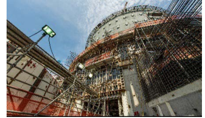
Vogtle Unit 3 containment building under construction. (Courtesy of Georgia Power/Southern Company, July 2018)
